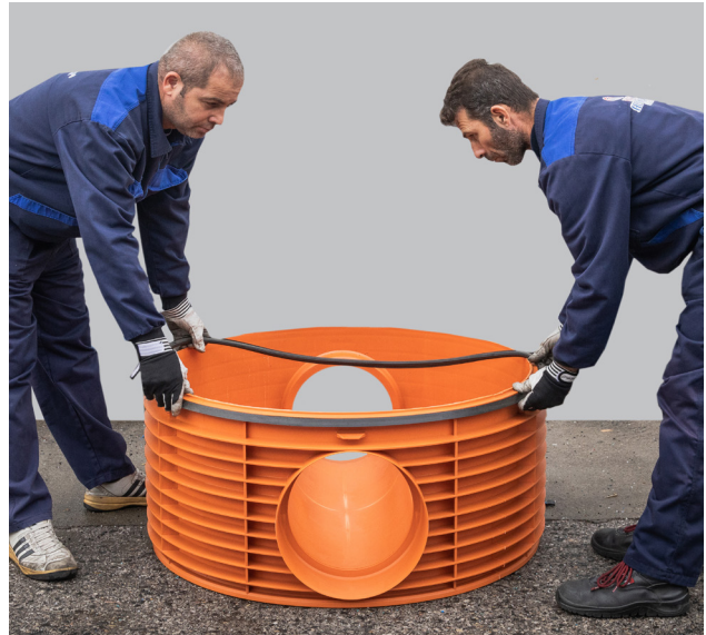
Installation of rubber
