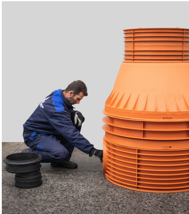
Lubrication for third rubber and preparation for cone installation
