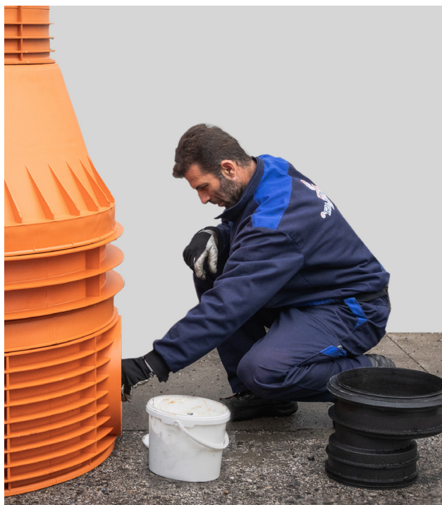
Preparation for side connection with reducer
