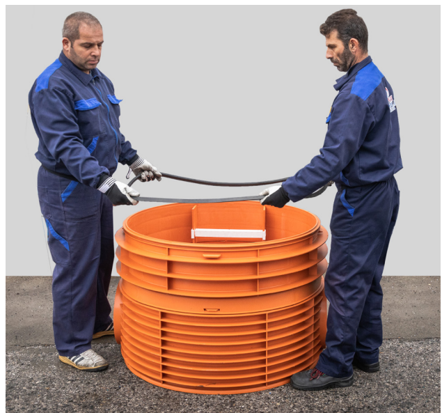
Preparation for installation of second extension, lubrication for second rubber and second extension
