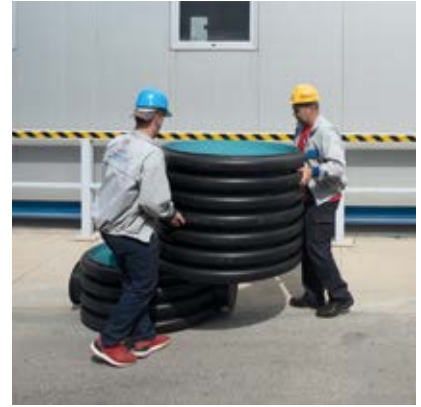
Above the bottom is placed the body from the ribbed tube, in a properly made groove for good setup with the bottom.
