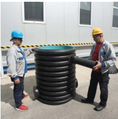
Complete assembly of the socket in the manhole's body.
