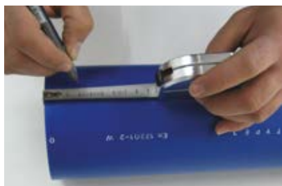
Measure and mark the pipe
