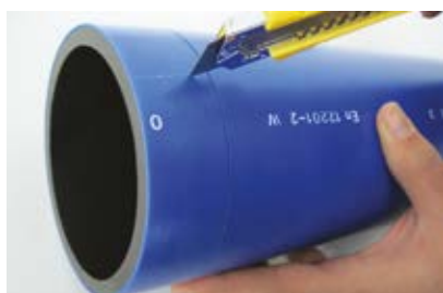
With scalpel make a cut on circle of top layer
